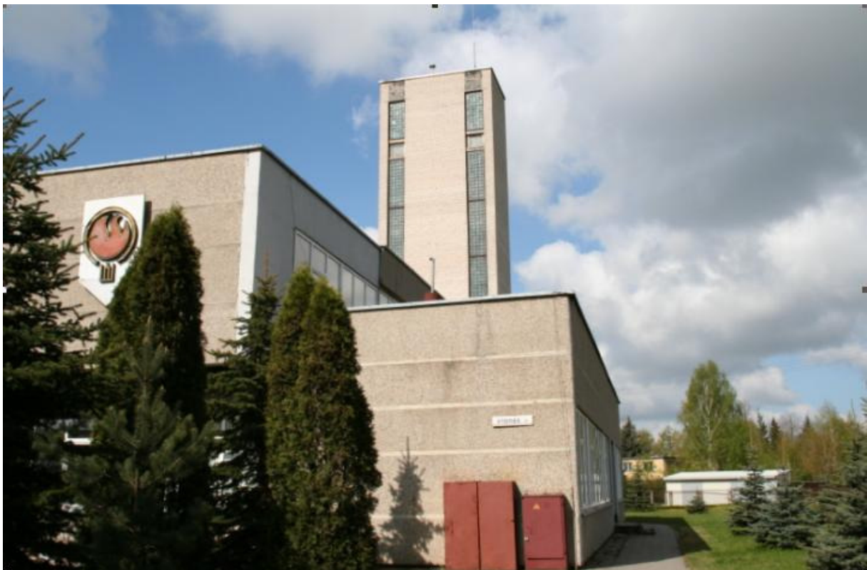
Fig. 3. GPS antenna on the roof of fire station tower
