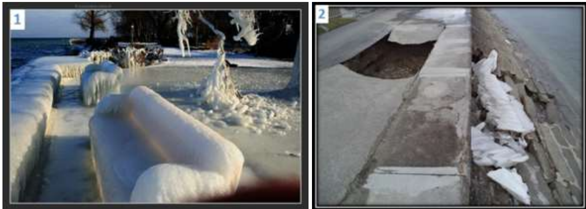
Fig. 3): Ice shield on the shore in February (left) [4]. Collapsed ground after the melting of the ice in March 2018 (right).
