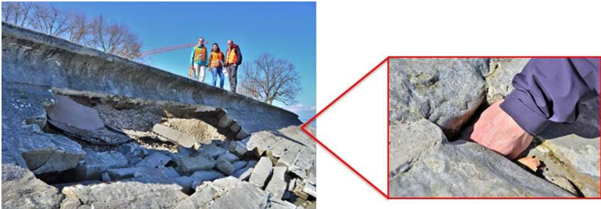
Fig. 4): Collapsed site near the promenade (left). Holes between the stones in the ramp (right).
