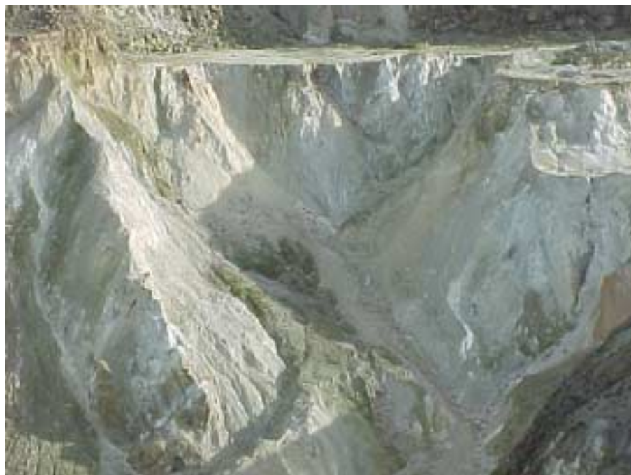
Figure No. 7 Photographic image of slope failure scar looking in an easterly direction.
