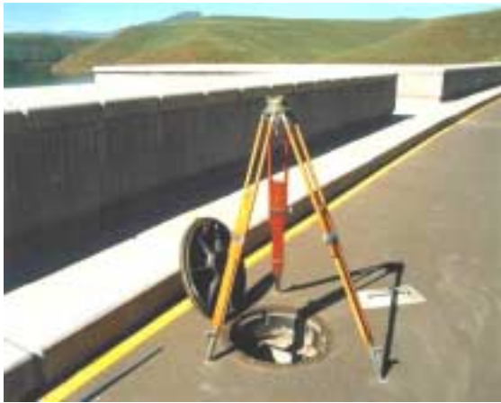
Figure 6 Crest Optical alignment monitoring point with tripod.
