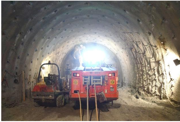
Figure 7. Tunnel construction site
