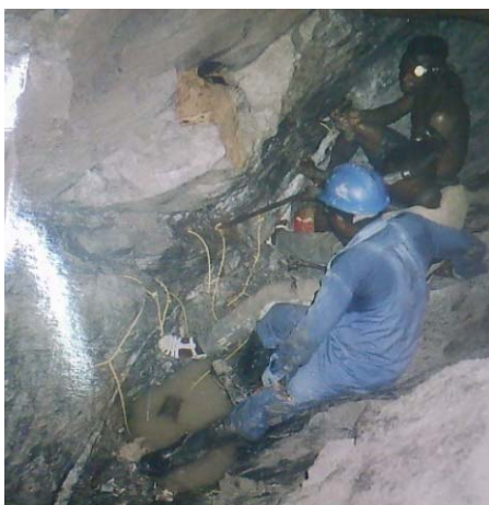
Figure 2.1 Small Scale underground mine in Tarkwa
