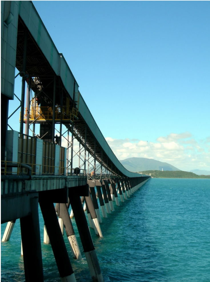
Figure 3: Civil engineering in the nearshore
