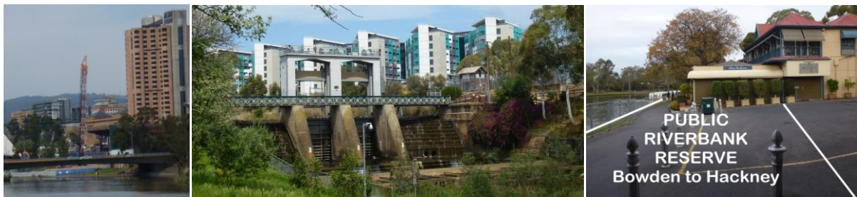
Figure 13: Riverbank development, Adelaide Park Lands: (left) Convention Centre expansion, (centre) Torrens Weir (foreground) / new hospital north elevation (background); (right) construction on public access reserve (Jolley’s Boathouse Restaurant). K. Henderson, 2015.
