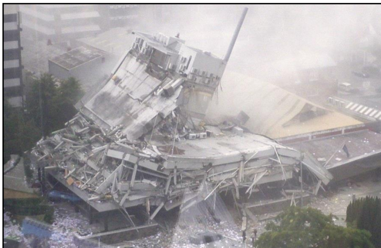
Figure 1: Collapsed PGC Building. Source: Fox and Associates.
