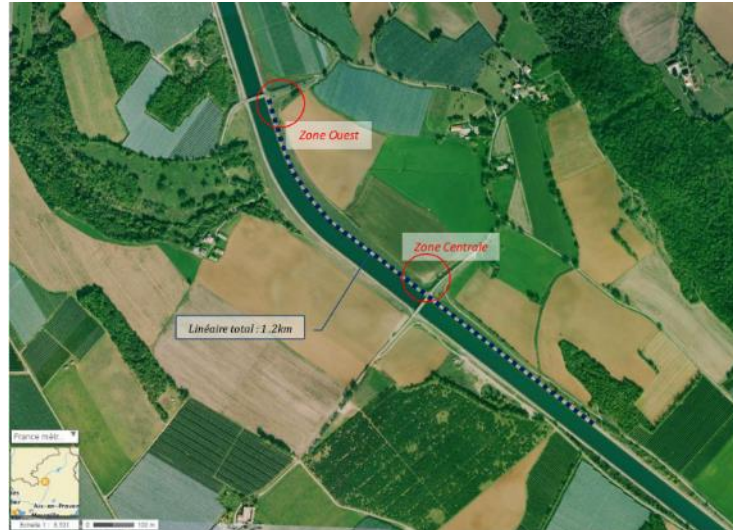
Figure 20: 1 km dike site for testing
