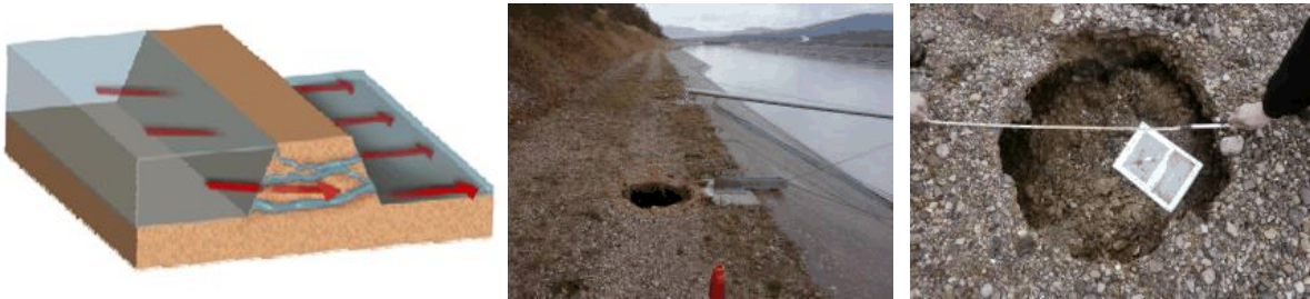
Figure 9: possible consequence of internal erosion
