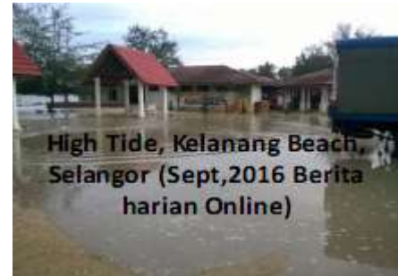
Flash flood due to high tide
