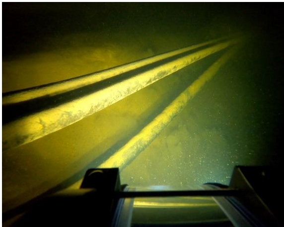
Fig. 11: ROV image of a pipeline crossing the spring pit
