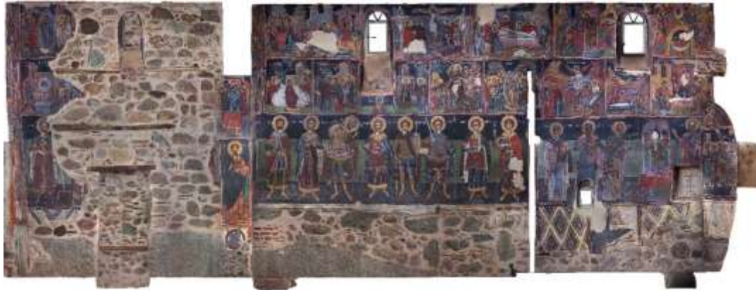
after the restoration works
